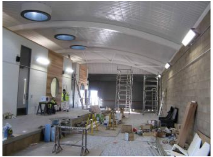
The interior of the building nearing completion on 5 th February.
