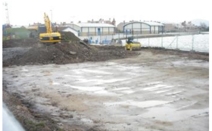
By 25 th March the building site looked like this.
